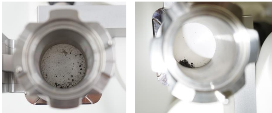
Left before flushing and right after flushing
